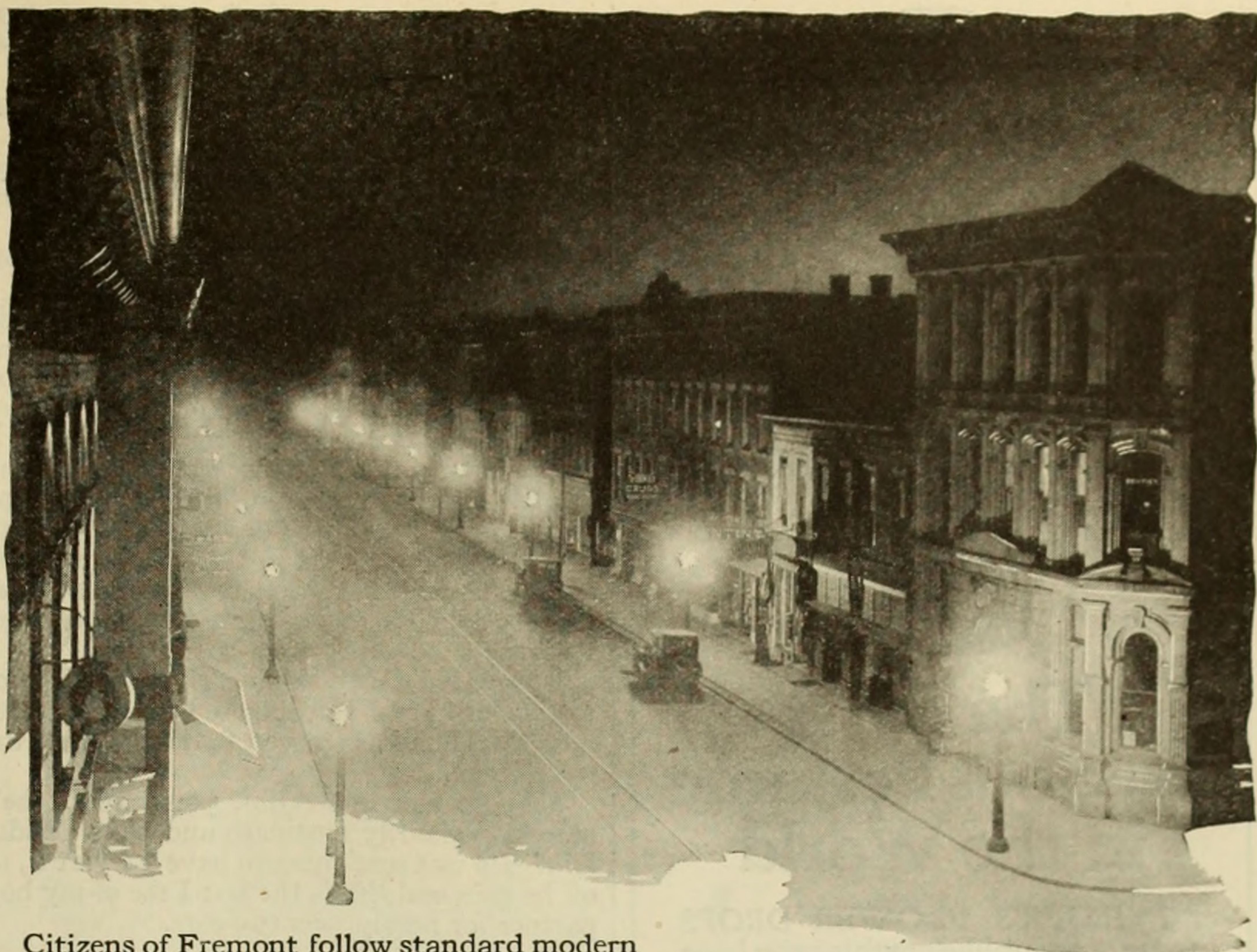
Citizens of Fremont follow standard modern lighting practice for business streets. The 600 candle-power lamps are spaced 80 feet apart.
