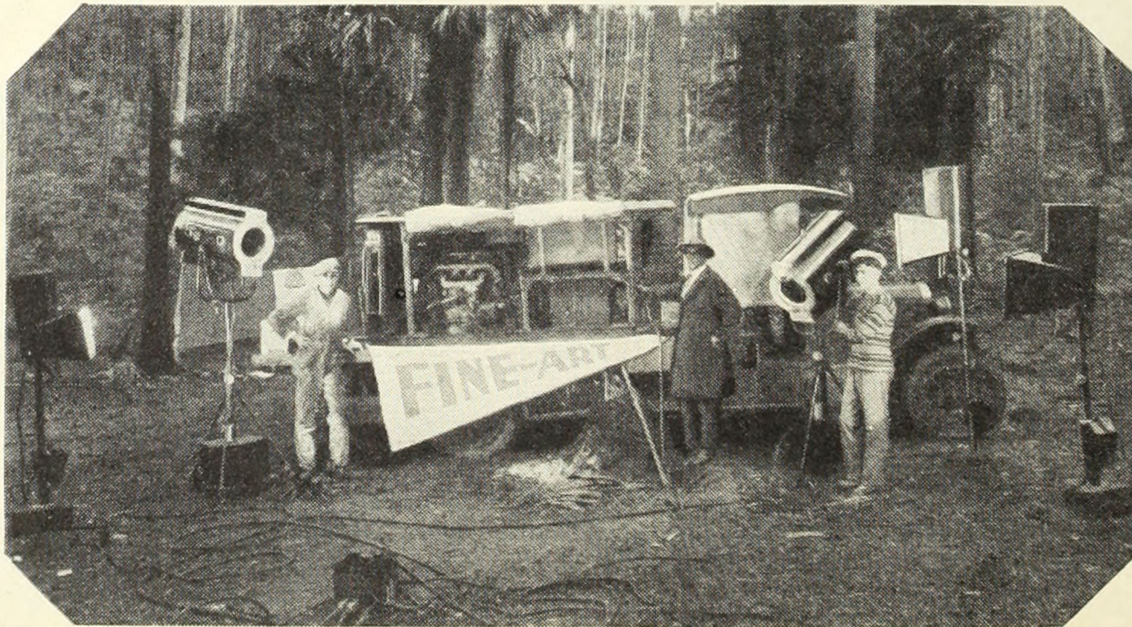
Here is part of the lighting equipment used in night sequences of "Pearl of the Pacific." The plant is 90 HP Petrol set direct, coupled to 450 amp. 110 Volt generator mounted on a truck
