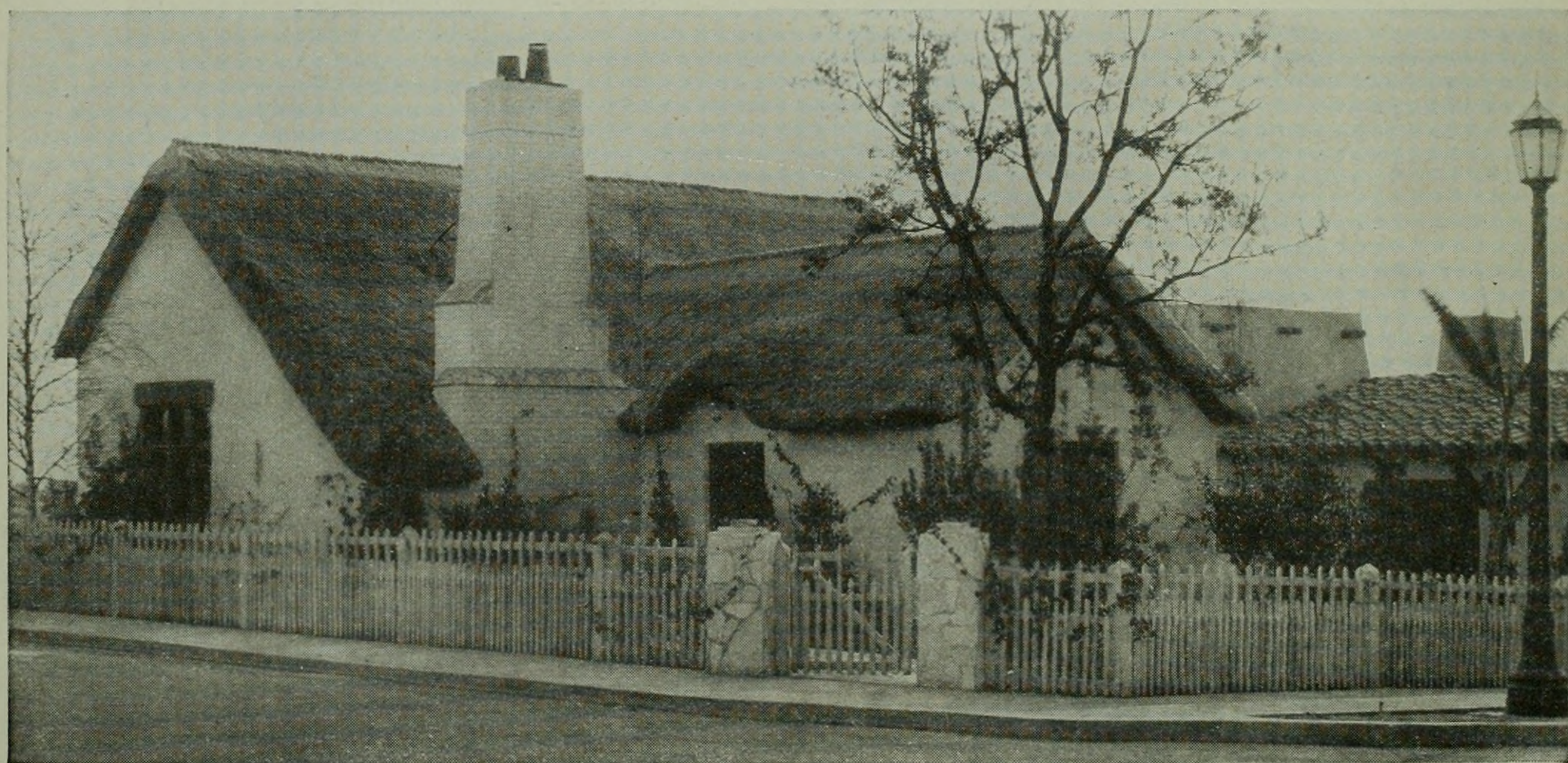
When Fox welcomed John McCormack to Movietone City, they built him this bit of old Ireland to make him feel at home. Every bit of thatch in the roof had to be fireproofed—not an old Irish custom
